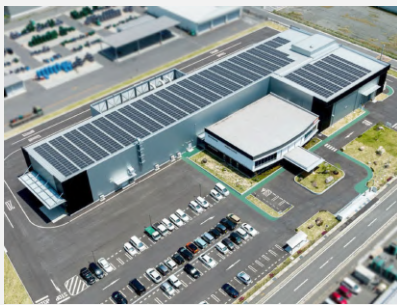
Solar panels on the Kurashiki Plant
