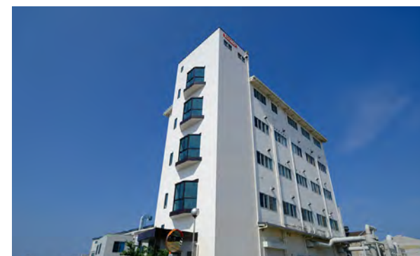
Thermal Spraying Technology R&D Laboratories
